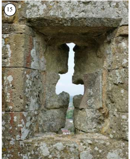
Figs. 12-15. The interior of the shell-keep. 12: Garderobe (inserted?) on the east wall (no dogleg). 13: Garderobe on the north wall (also seen in 14). 14: Looking west along the curious high-walled corridor to the entrance gatehouse. Probably a post-medieval 16 th -century addition. 15: One of two arrow loops on the top of the gatehouse.
