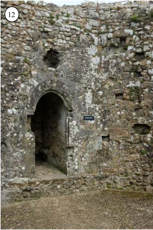
Figs. 12-15. The interior of the shell-keep. 12: Garderobe (inserted?) on the east wall (no dogleg). 13: Garderobe on the north wall (also seen in 14). 14: Looking west along the curious high-walled corridor to the entrance gatehouse. Probably a post-medieval 16 th -century addition. 15: One of two arrow loops on the top of the gatehouse.
