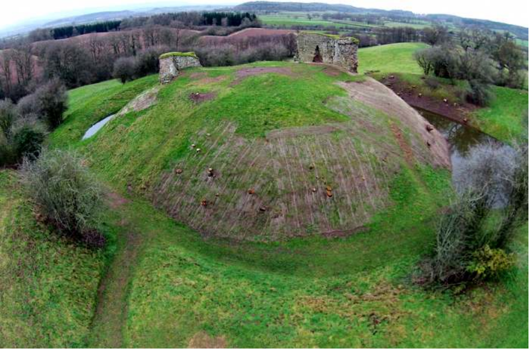
Fig. 1. Kilpeck Castle, Herefordshire. From the south-east. It has two remaining sections of walling, the largest to the north, and one to the west. Image courtesy of CBS Conservation ( cbsconservation.co.uk ) who undertook major consolidation works to stabilise the structure in 2013.
