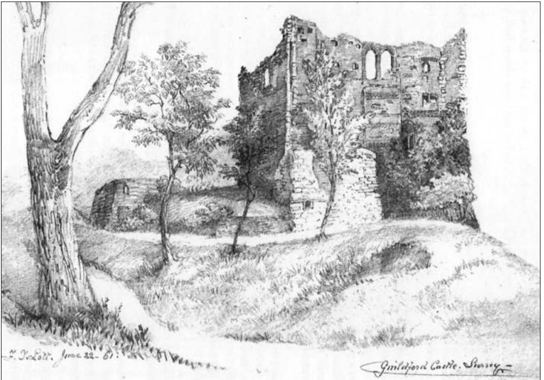
BELOW: Fig. 4. Drawing of the motte with its buildings in 1861 by F. T. Lott, showing some remaining parts of the shell wall. Looking toward the shell keep from the south. In front of the keep there is perhaps a latrine chute just below a string course (not seen on fig. 1). Courtesy of Guildford Museum, (Catalogue no. G.7785).
