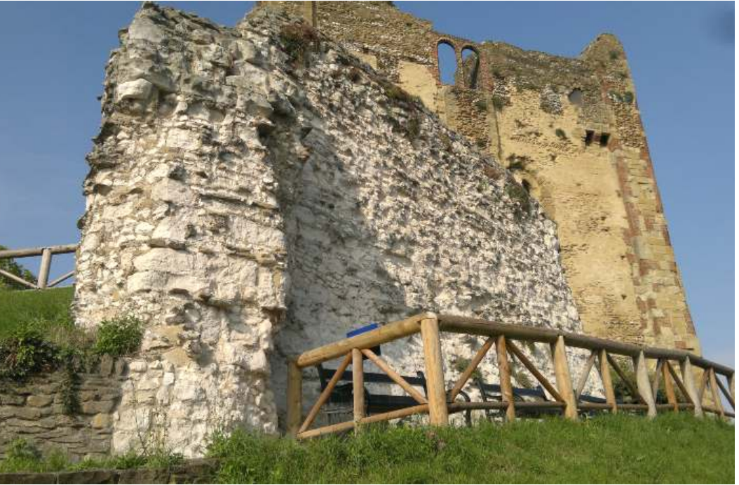
Fig. 1. Guildford Castle shell wall and keep, from the south. The shell is built of local chalk but the keep of Bargate stone. The image 'Guildford Castle (2)' is by Richard Nevell. Licensed under CC BY-SA 3.0 via Wikimedia Commons. Reproduced with thanks.
