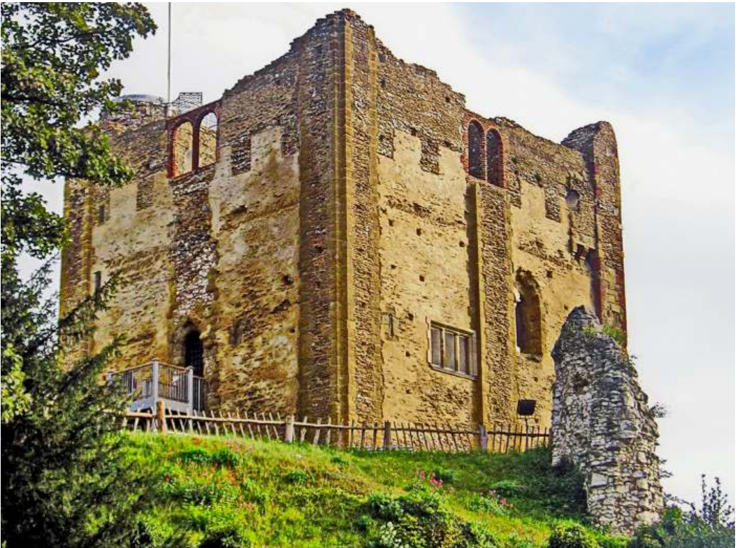
BELOW: Fig. 9. Fragment of the shell wall, (buttress or turret), and rectangular keep to rear, from the south-west (cf. fig. 1). The shell wall fragment appears to partly revet the motte.
