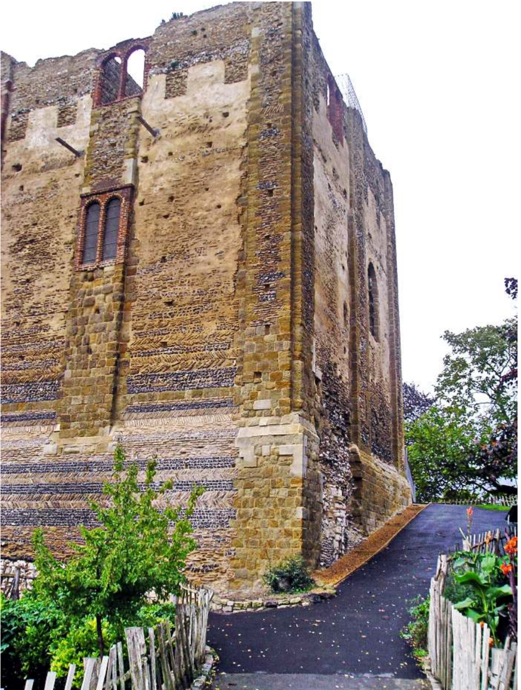
Fig. 10. The scar on the north wall of the rectangular keep where the shell wall joined. The path follows the line of the original entrance. The east wall of the keep is 10ft lower than the west, The keep entrance is on the west side. The keep was heightened - note the crenellations of the first build, picked out in render.
