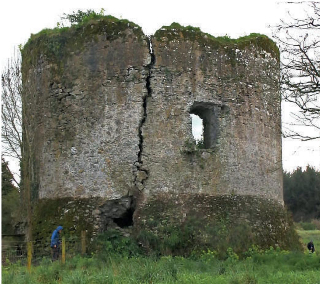
*Inchiquin tower, currently in poor condition. View from the north. With an internal width of 10m and an external width of over 16m this puts it in the same league as the Pembroke tower in terms of its diameter and wall thickness at least. (7.7m x 19m inc. batter).*
