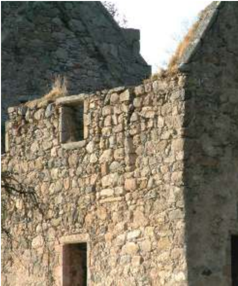
Fig. 8. Detail, taken in 2003, showing the blocked up doorway on the second floor of the tower.
